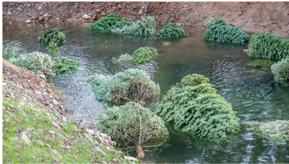
TREES FOR TROUT: Trout Unlimited and RI DEM team up to help control water flow in rivers and erosion through the strategic placement of Christmas trees. (Submitted photo)
